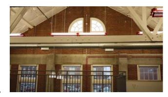
installation of storm windows and the reconstruction of a roof monitor, along with new mechanical and electrical systems. All work conformed to historical building restoration standards.
